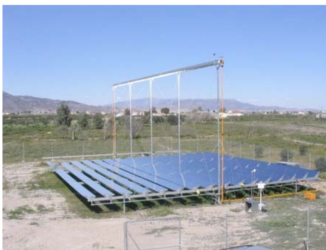
Figure 11: Picture of a concentrating solar field (courtesy of Novatec Solar)
