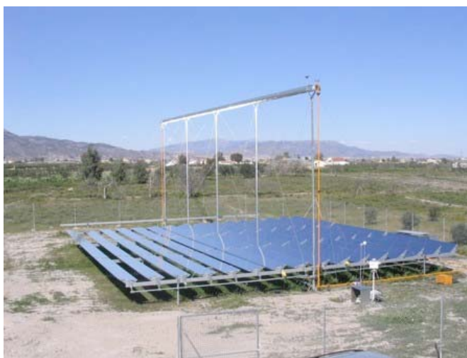
Figure 6: Picture of a concentrating solar field (courtesy of Novatec Solar)
