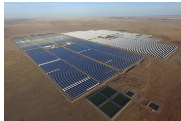
XiNa Solar One, parabolic trough collector plant with storage developed by Abengoa in South Africa.
