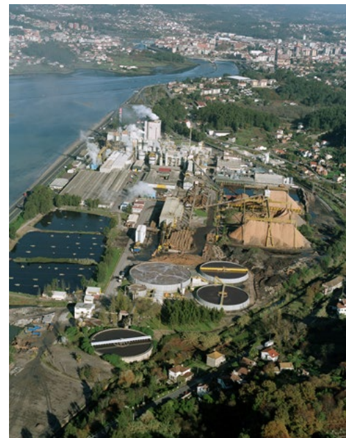
Industrial water treatment plant in Ence Pontevedra developed by Abengoa.
