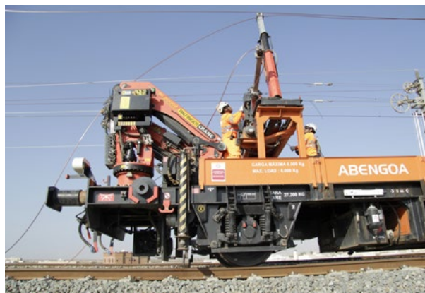
Image of the Mecca - Medina project works in Saudi Arabia.
