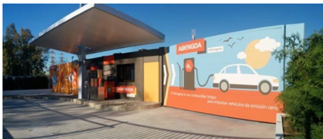
Hydrogen service station.
