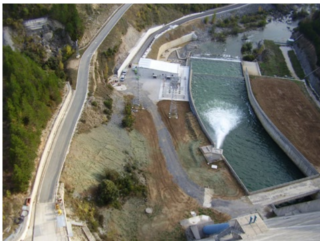
Power plant developed by Abengoa at the foot of the Itoiz dam.
