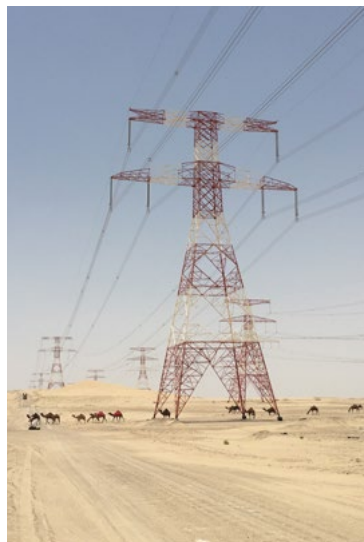
Abengoa has carried out the construction of the Faya-Shamkha power line.
