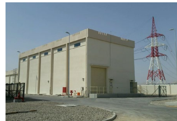
Abengoa has put the 132/33 kV Al Dreez substation into service.
