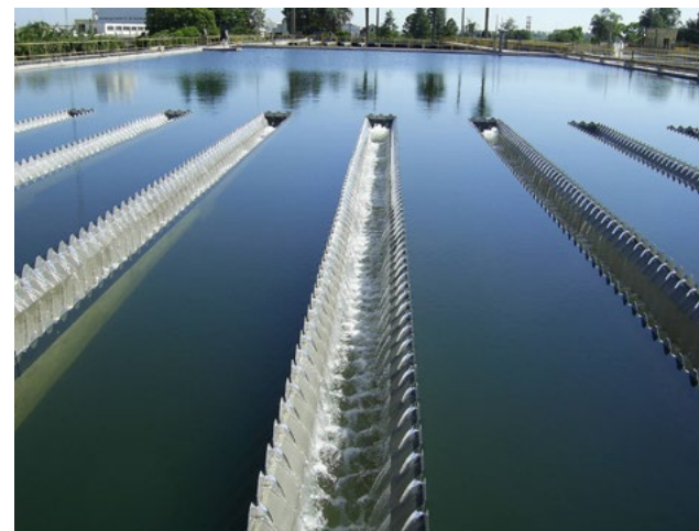
Detail of water treatment plant carried out by Abengoa.
