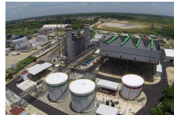
Aerial view of the A3T efficient cogeneration plant, which is being developed by Abengoa in Mexico.
