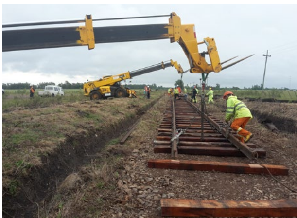
Abengoa's railway rehabilitation works in Uruguay.
