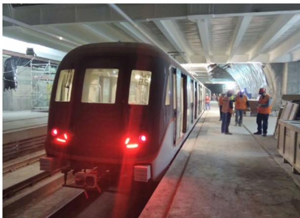
Line 6 of the Chile Metro.
