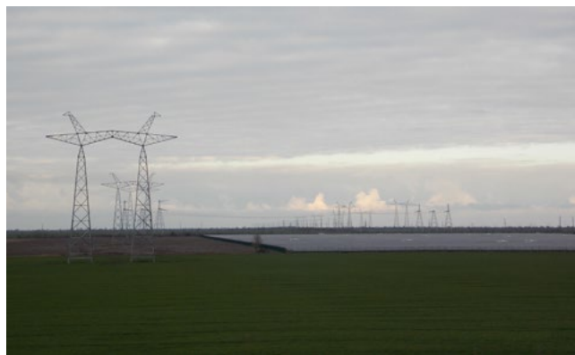
In Ukraine, Abengoa continues with construction of a 765 kV line along 187 km.
