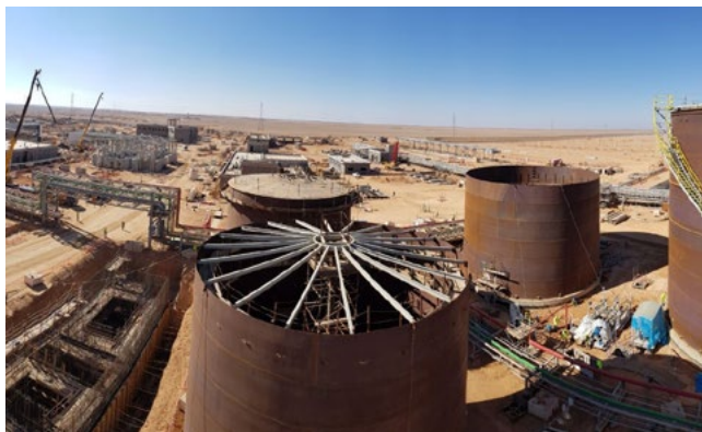
Image of the Waad Al Shamal works.
