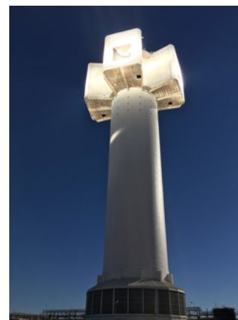
Image of the tower and receiver of Khi Solar One, in South Africa.
